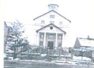
The fence and gate are now finished at Efrata church!
